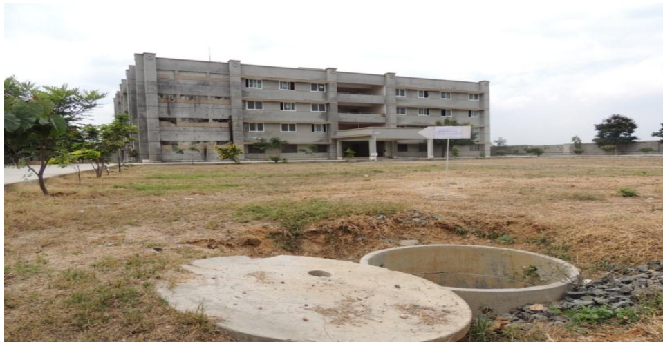
Rain water harvesting pit at in front of boys hostel
