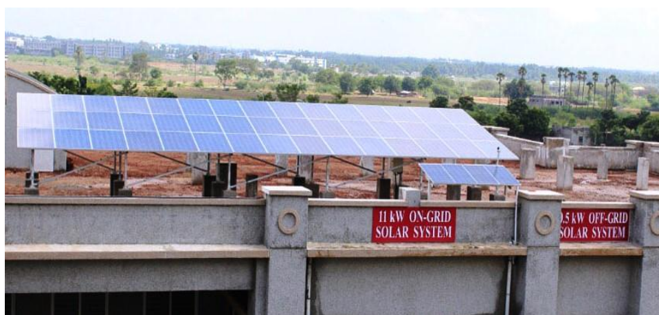
11 kW “On-Grid” Solar energy harvesting system
